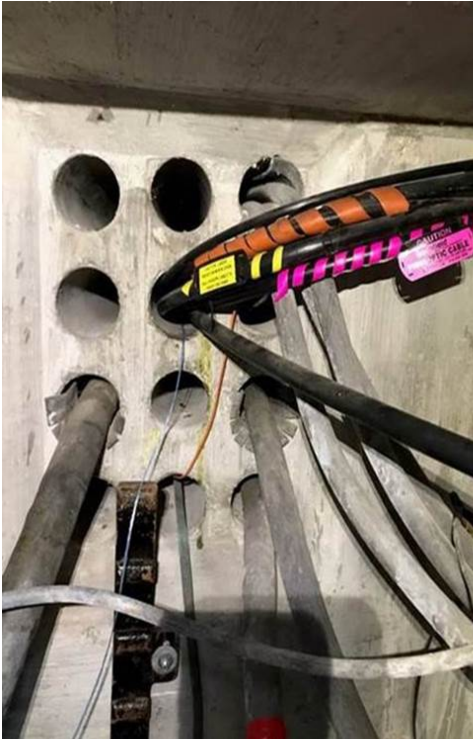
Typical Photo 3. Cable chamber with labelled cables
